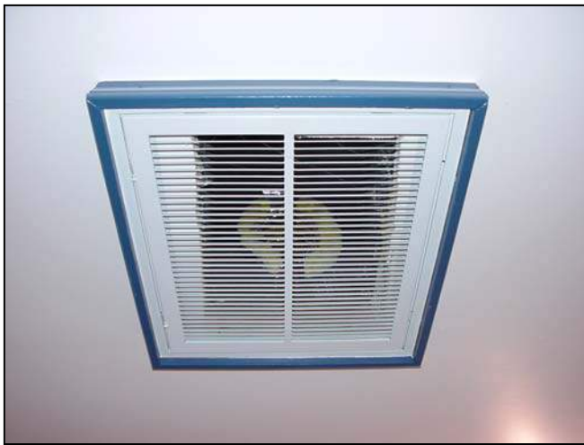
Figure 4.6a — Silent duct boot, grille closed
