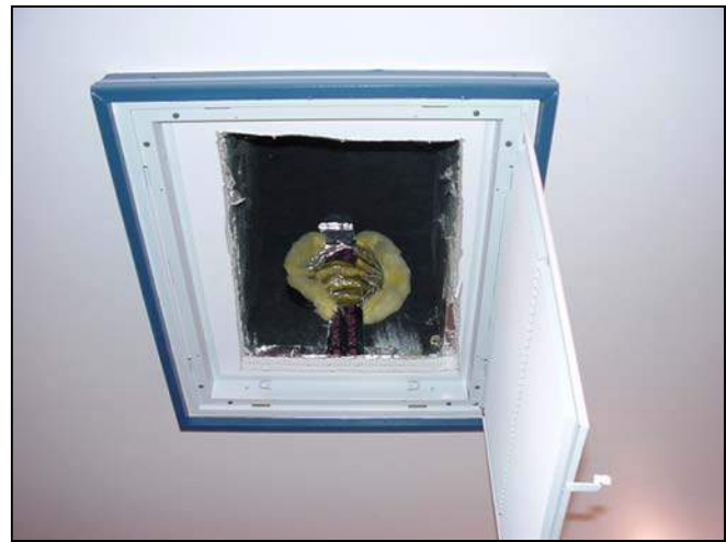
Figure 4.6b — Silent duct boot, grille open
