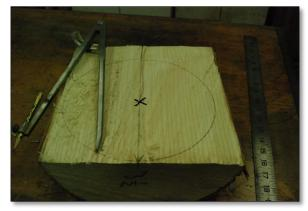
Figure 10: Draw the circle for the blank as shown. Be sure to note where the center of the blank is located by drawing a large "X" with a marker. It is often hard to find the center point hidden under the Anchorseal.
